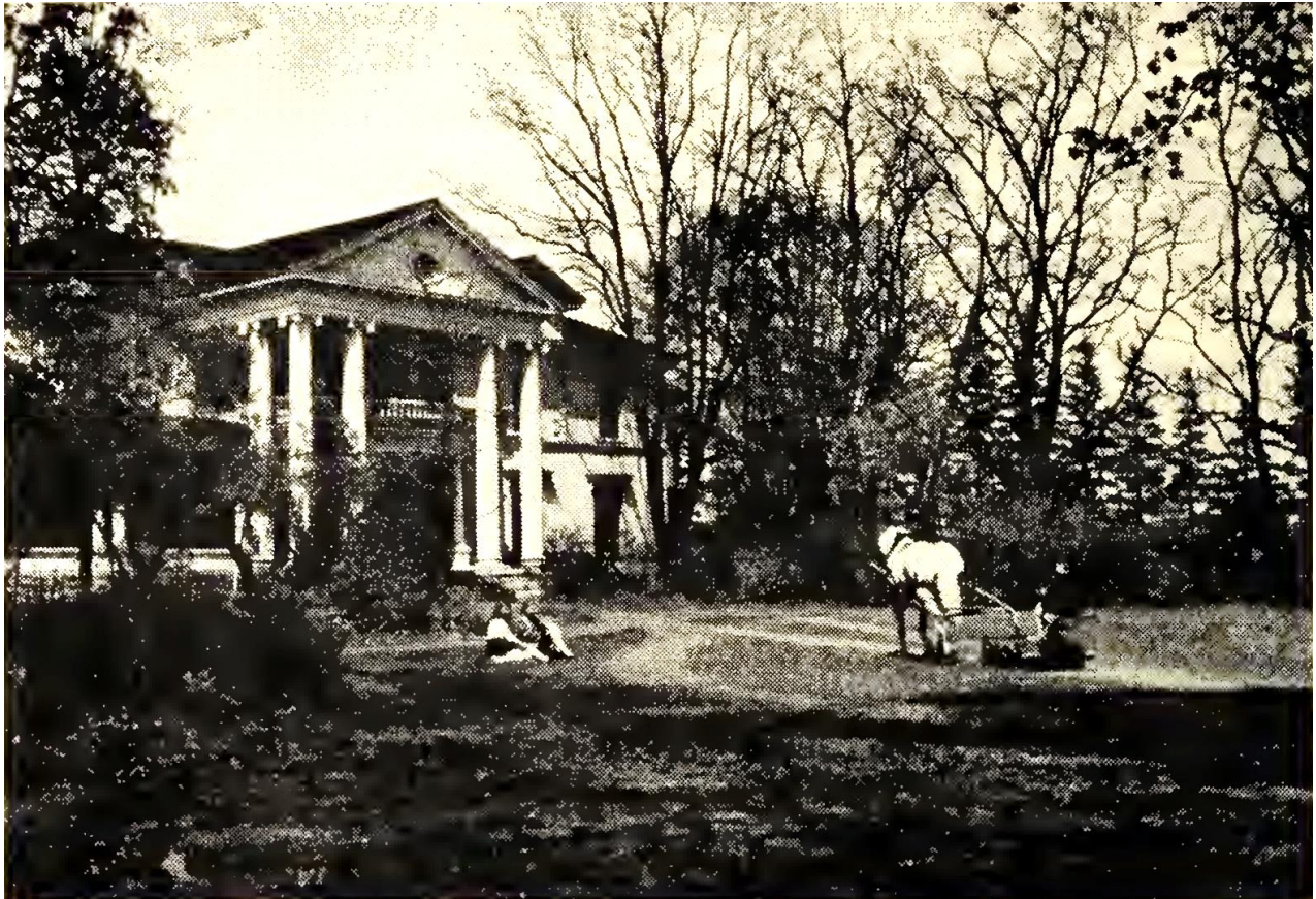
STRATHMORE – one of two fine residences acquired by the Department of Reform Institutions to serve as a Training School for Girls under the age of sixteen. These spacious dwellings with beautifully landscaped grounds are located in Cobourg, Ontario.
