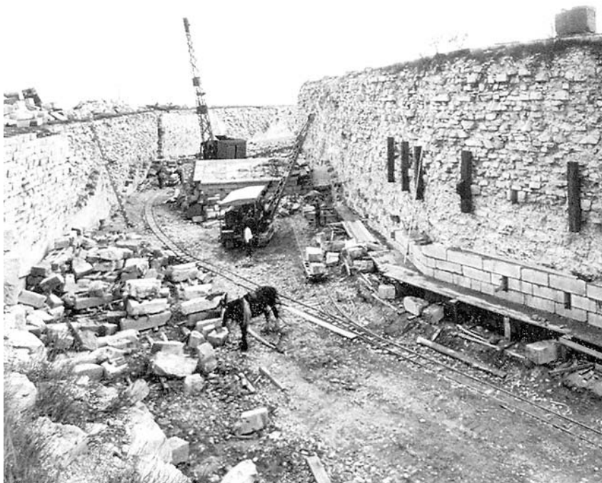
Here is Fort Henry's limestone ditch being constructed in 1832
