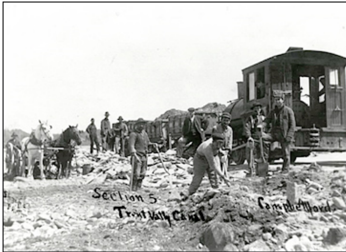
Construction crew working on the canal at Campbellford Courtesy Dennis Carter-Edwards, Trent-Severn Waterway
