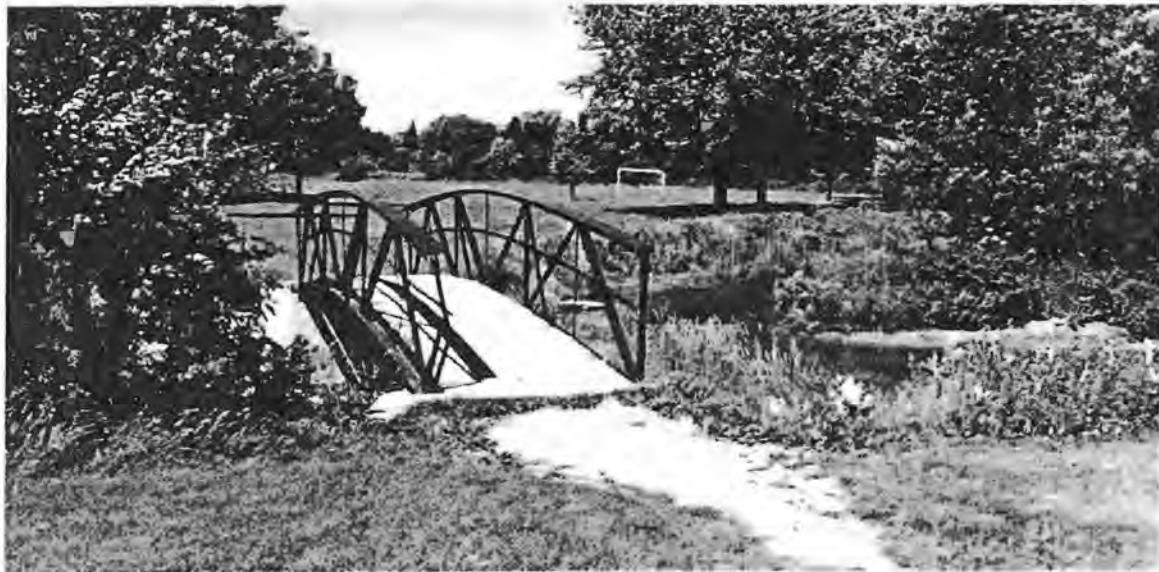
Figure 1: Bridge at confluence of rivers in Rotary Park. Photograph © John Jolie 2004
